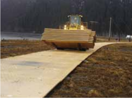
The mat systems are used for a variety of applications such as temporary roadways.
