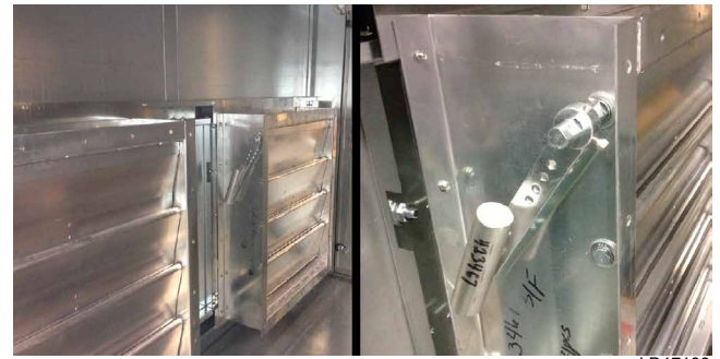
FIGURE 6 - COUNTERBALANCE LOCKED INTO PLACE FOR SHIPPING
