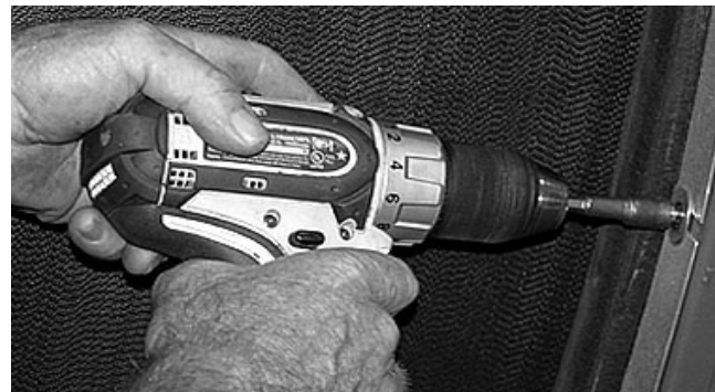
FIGURE 75 - LOOSEN SCREWS BEFORE ADJUSTING SEALS
