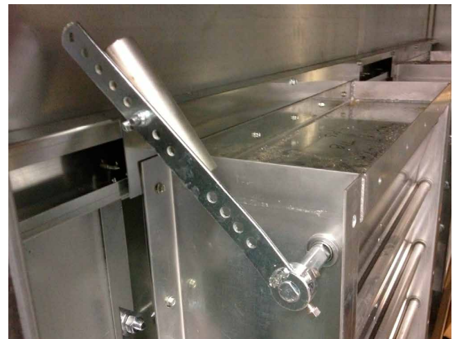
FIGURE 7 - COUNTERBALANCE UNLOCKED FOR START-UP
