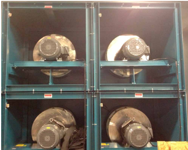
FIGURE 9 - BACK OF A 2X2 FAN ARRAY
