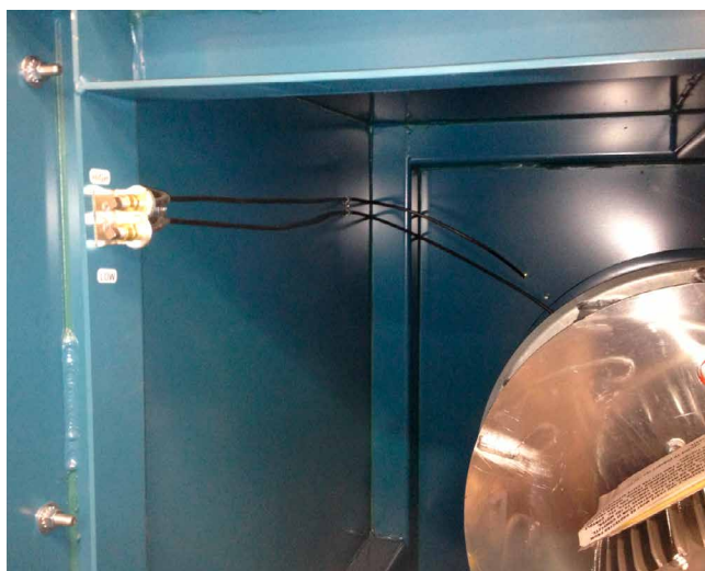
FIGURE 12 - HIGH AND LOW CONNECTIONS AND ASSOCIATED TUBING FOR FAN MOUNTED AIR MONITORING SYSTEM
